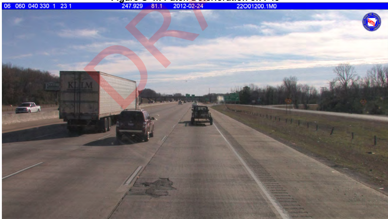
Figure C-4f. Patch Deterioration on I-40
