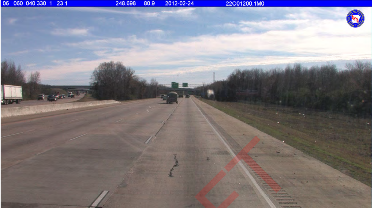
Figure C-4g. Linear Cracking on I-40
