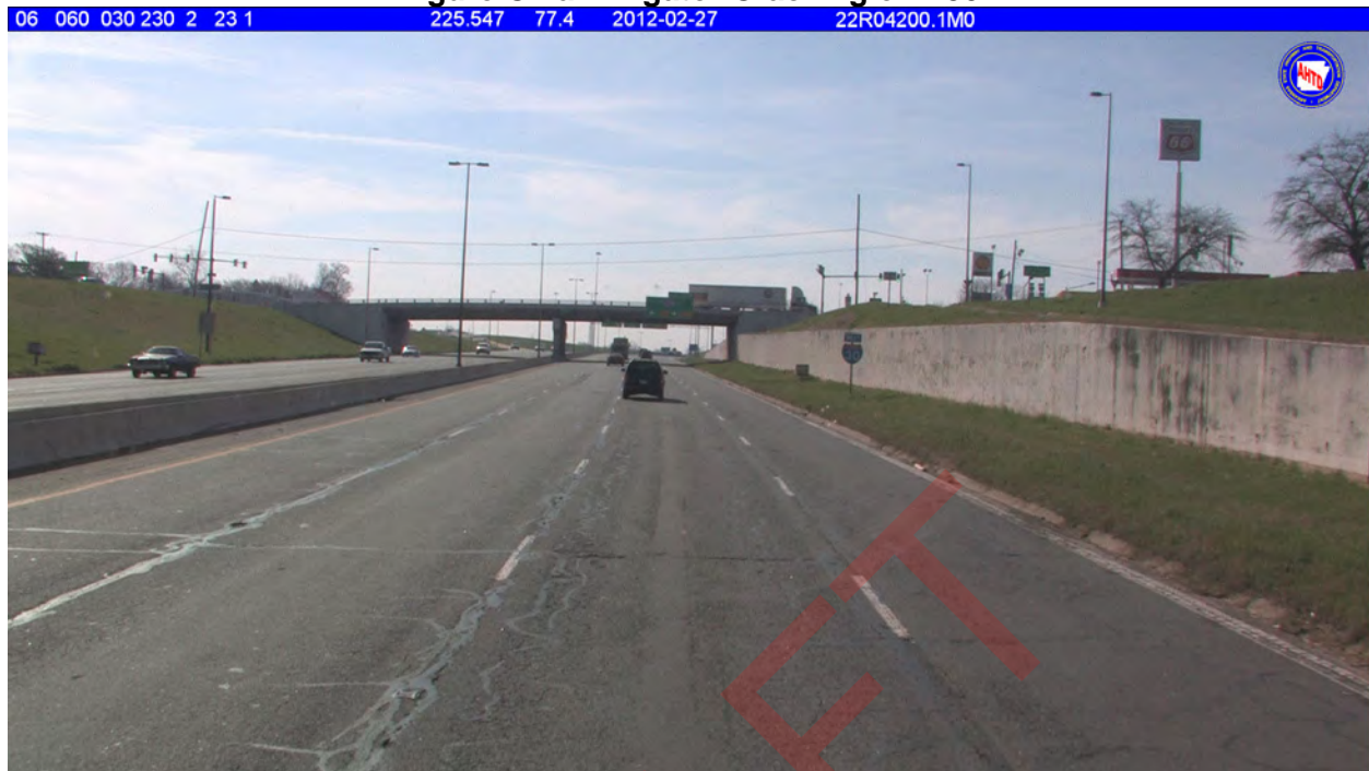
Figure C-4b. Joint Reflection Cracking on I-30
