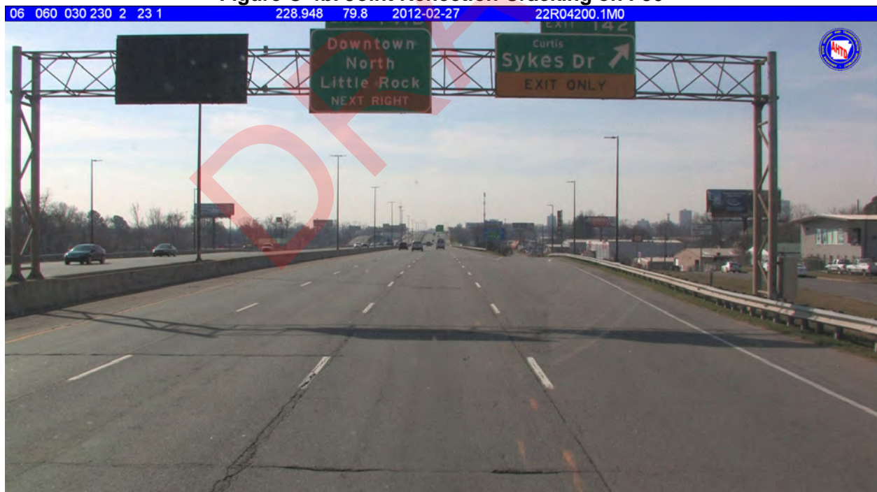
Figure C-4b. Joint Reflection Cracking on I-30
