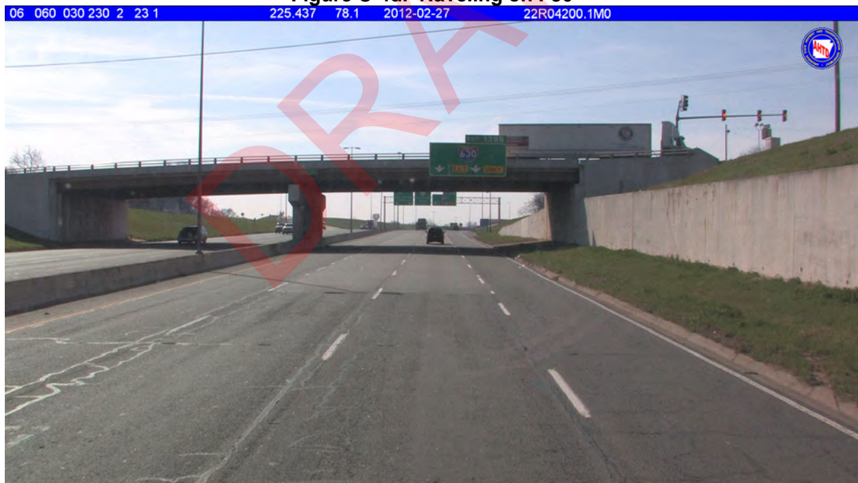
Figure C-4d. Raveling on I-30
