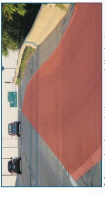
Deficiencies include ramps lacking recommended lane lengths.
