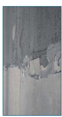
Deficiencies include pavement cracking, patch deterioration, joint separation, and raveling.
