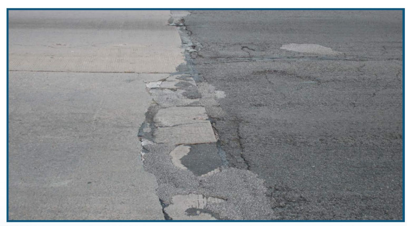
Deficiencies include pavement cracking, patch deterioration, joint separation, and raveling.
