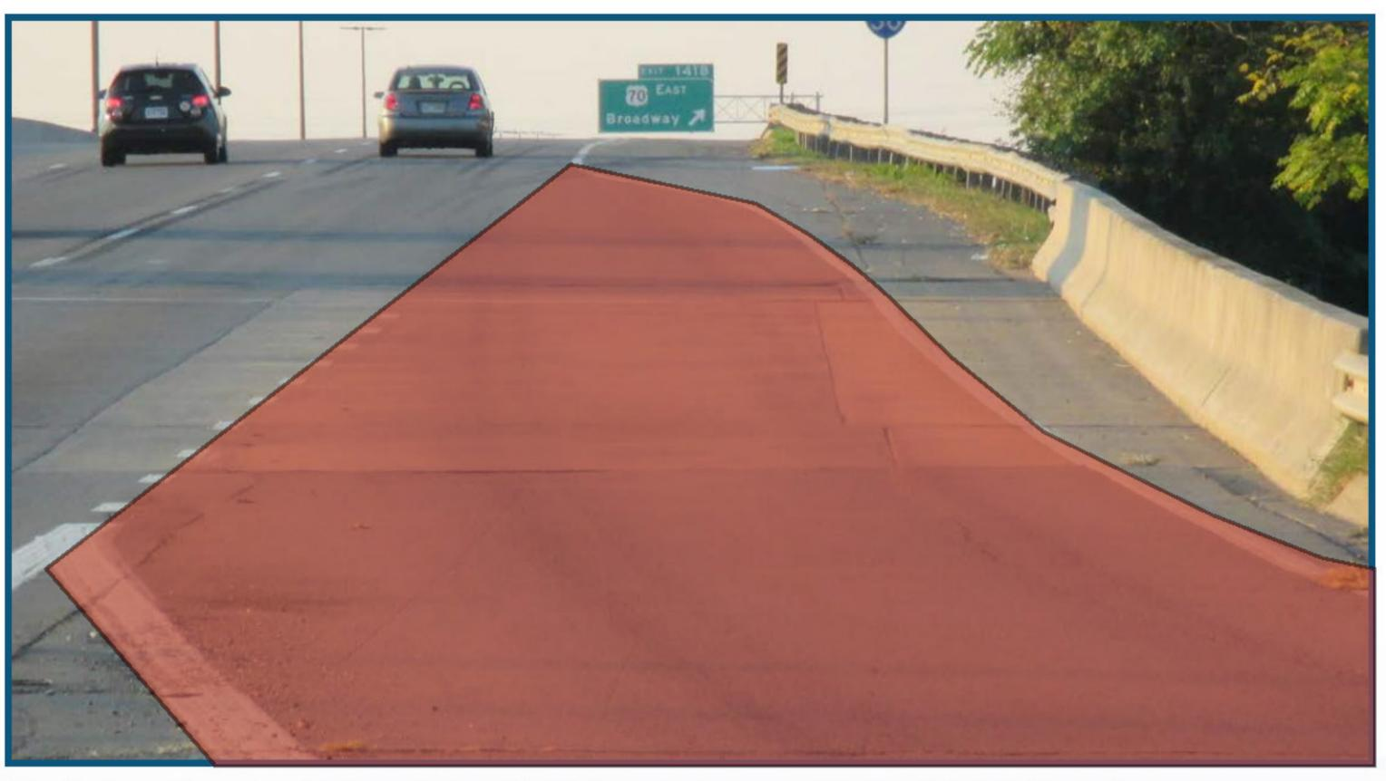
Deficiencies include ramps lacking recommended lane lengths.
