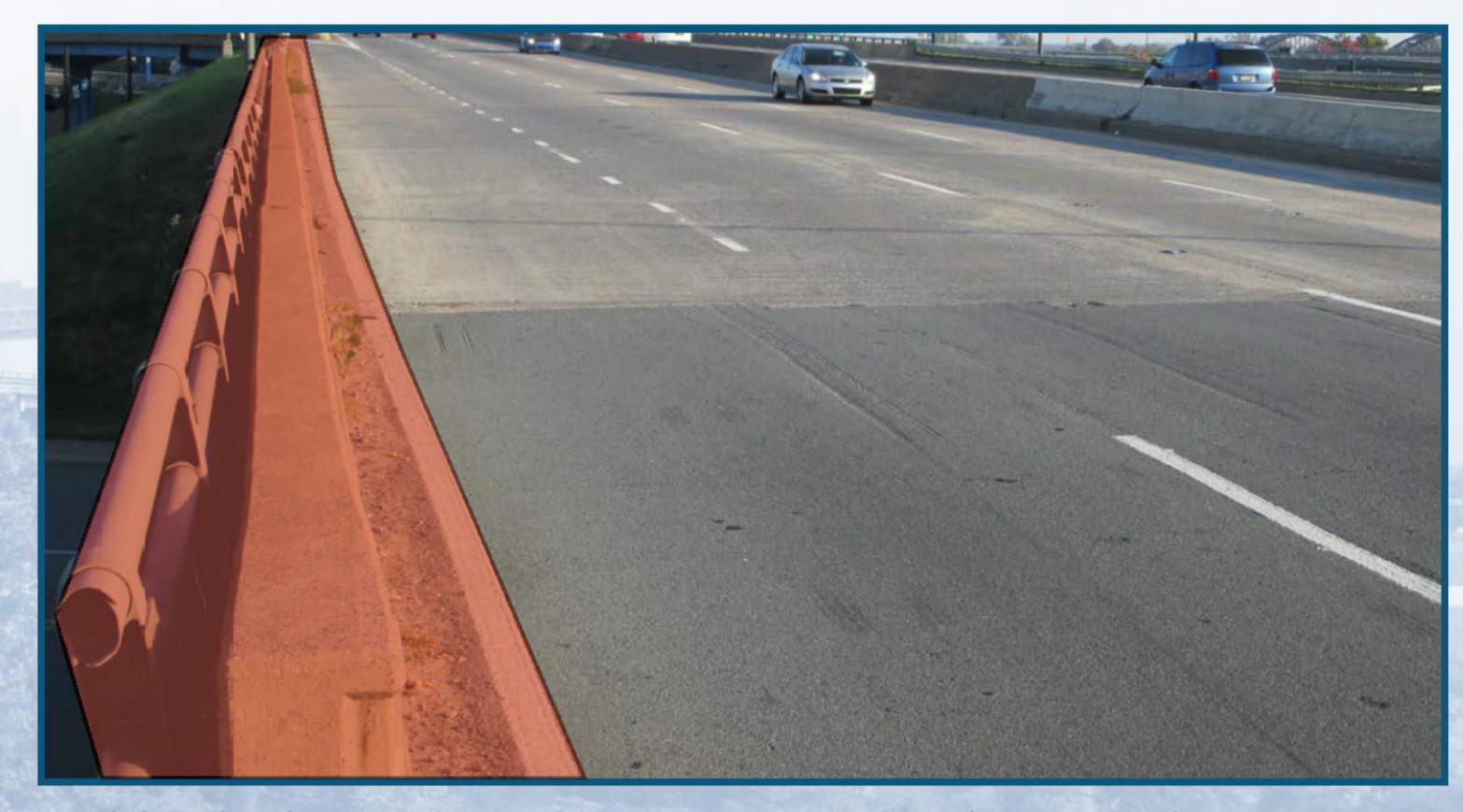
Deficiencies include lack of adequate shoulder widths on bridges.
